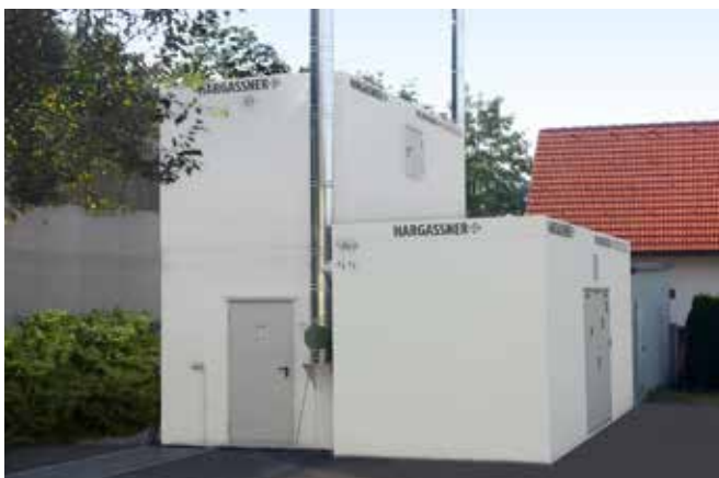
Triple-floor heating module in a catering operation.
